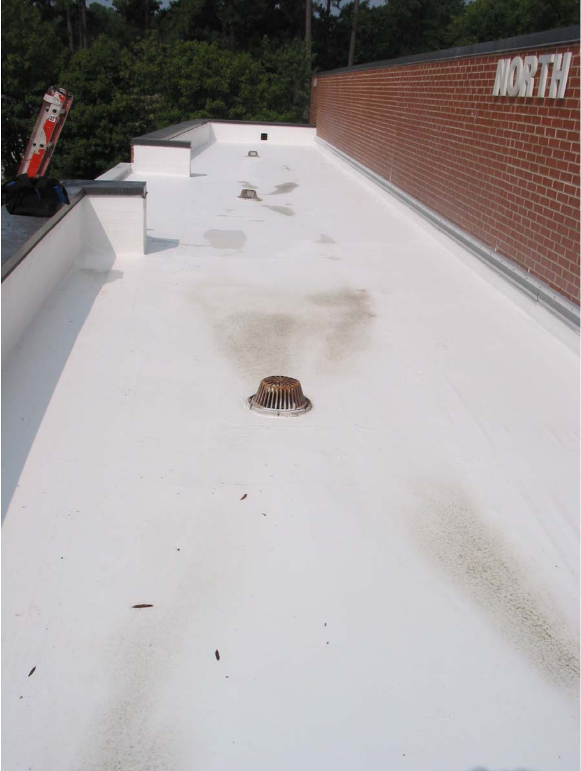
Details around parapets, crickets and drains
