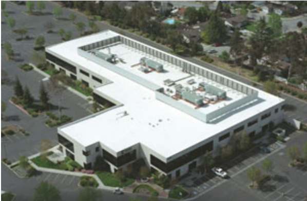
Photos courtesy of National Coatings Corp., Camarillo, Calif.
