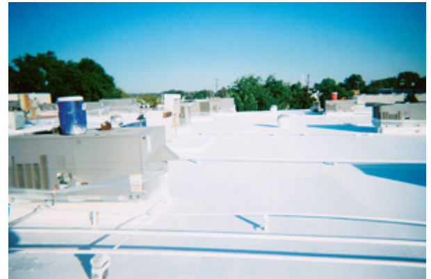
The topcoat process and HVAC protection
